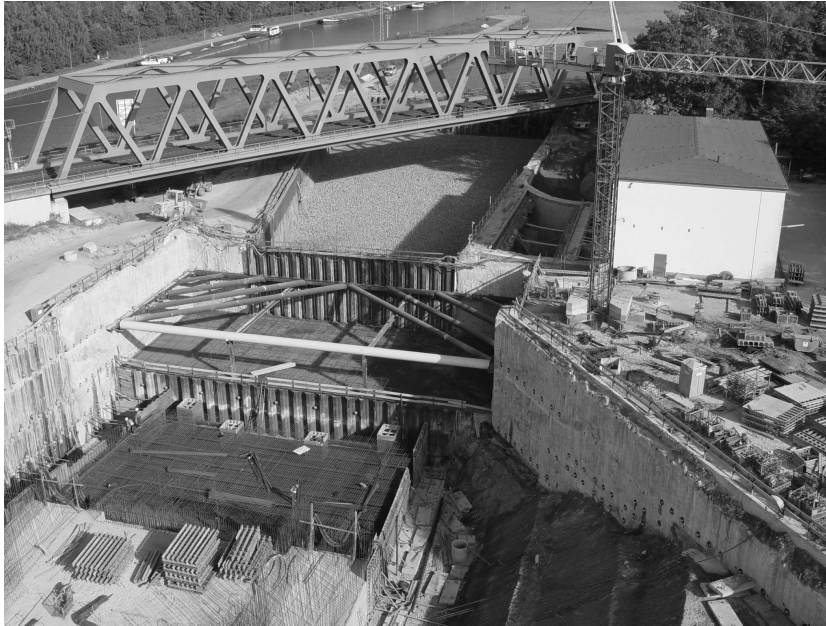
Figure 9.2: Strutted and back-anchored Sülfeld excavation near the railway bridge. The section left hand side of the channel's centerline is shown in Figure 9.3.
