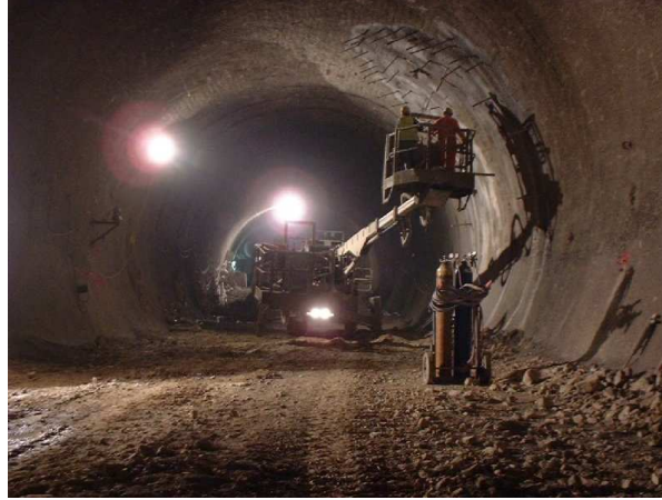
Figure 8.12: Steinhaldenfeld NATM tunnel before concreting the inner liner.
